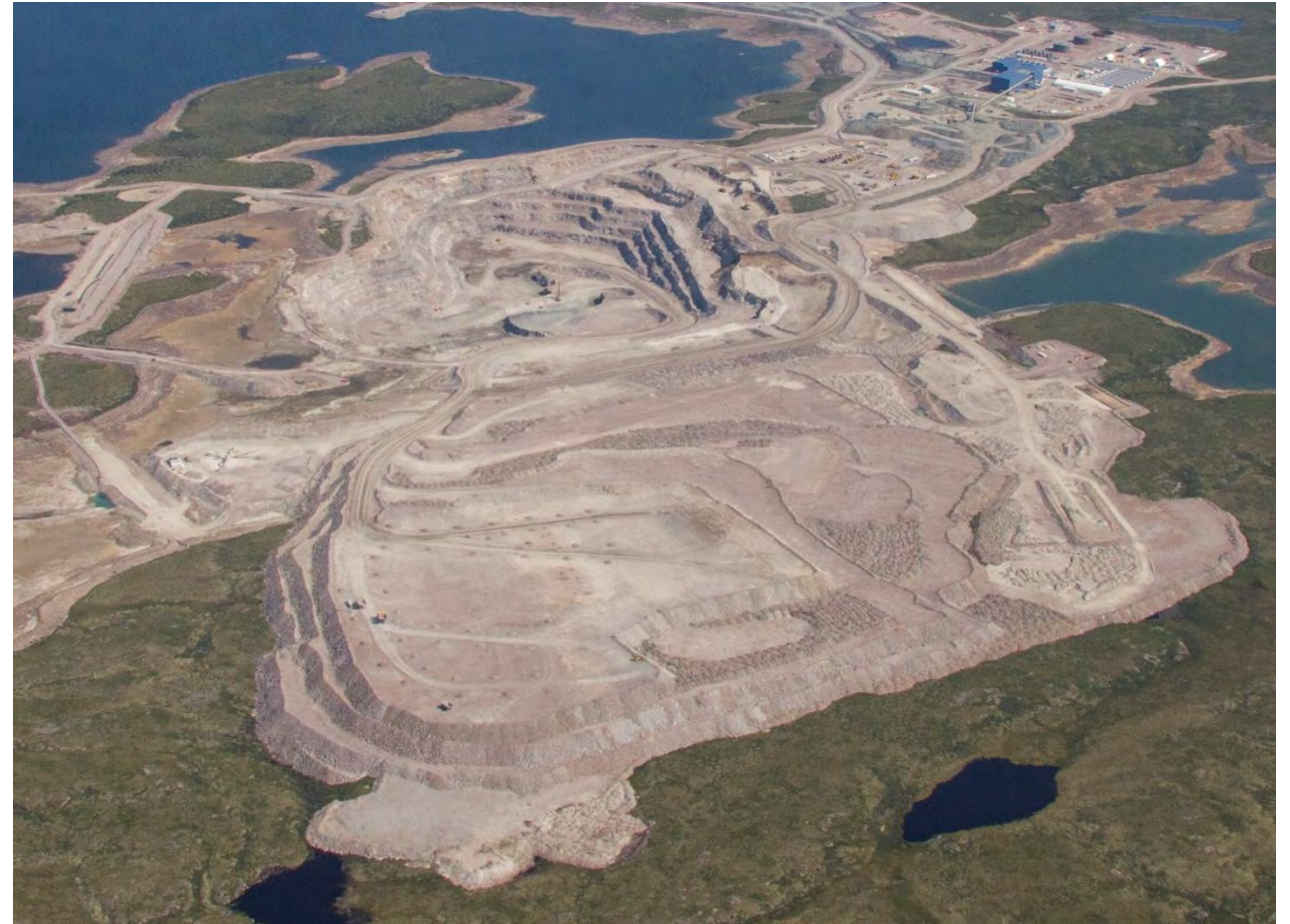
Foreground: South Mine Rock Pile in development; Background: 5034 Pit and Mine Site
